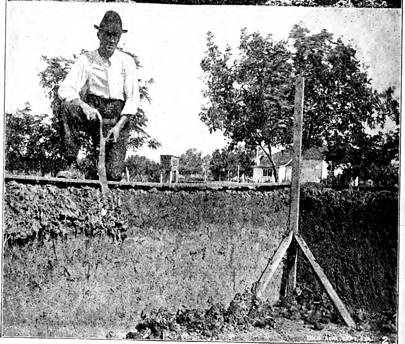
PLATE I.—1. Tramping the Abobe. 2. Trimming edge of wall with hay knife.
